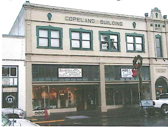
Figure 15. Non-Industrial Building, Flat Roof Behind Parapet Wall
